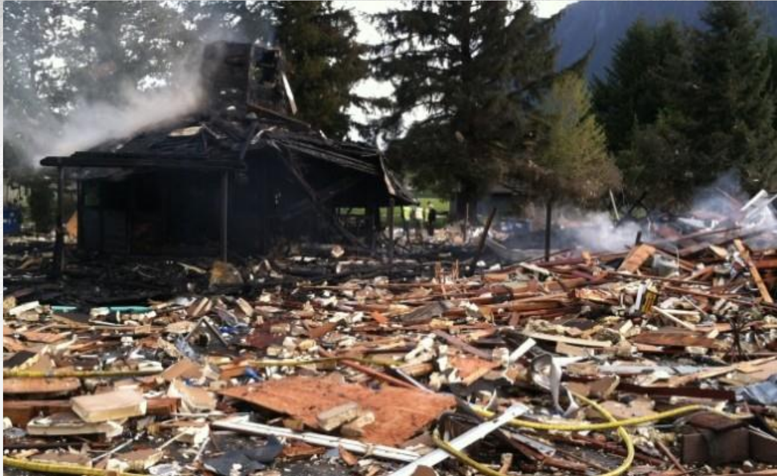
April 25, 2014, North Bend natural gas explosion
